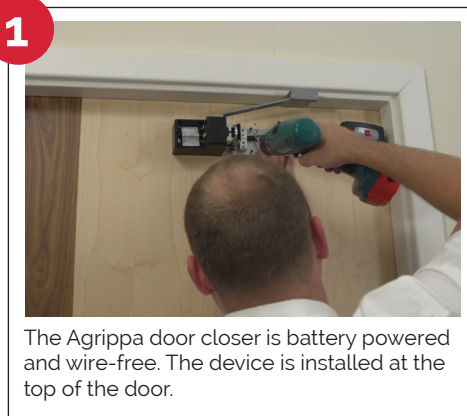
Using 'listen and learn' technology, the device learns the sound of the building's fire alarm.
